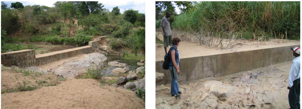
Figure 4. SASOL sand storage dams in Kitui (pictures field visit July 2006, P. Droogers & A. van Loon).
