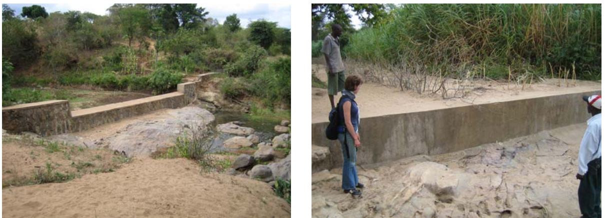
Figure 6. SASOL sand storage dams in Kitui (pictures field visit July 2006, P. Droogers & A. van Loon).
